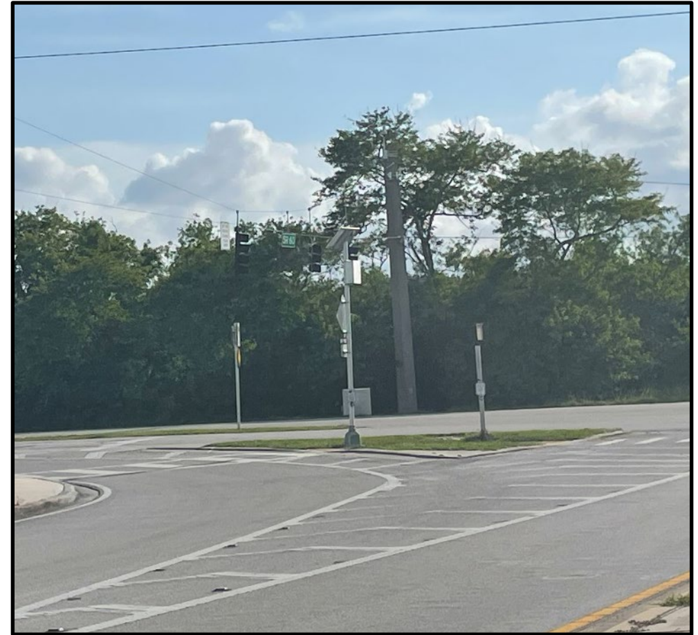
Intersection of SR 60/Merrill P. Barber Bridge at SR 60/Indian River Boulevard looking west (pre-construction)
